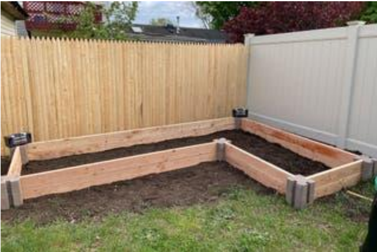
Jasmine used 50-pound weights to ensure the glue between her Oldcastle planter wall blocks dried securely. Photo: Jasmine Khoury
